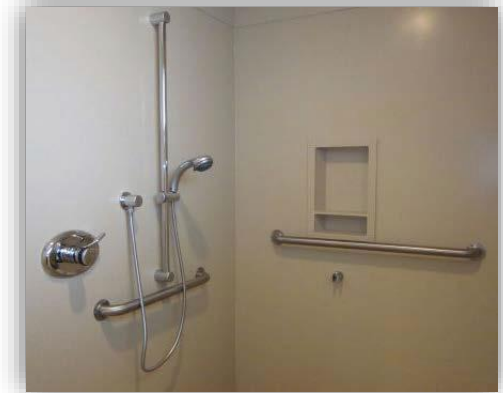
Grab Bars and Shower-head Extension
